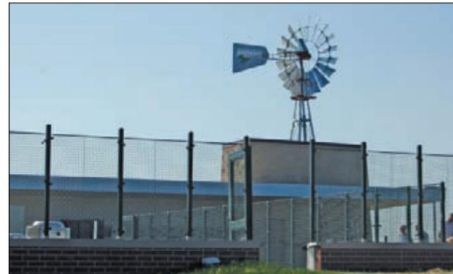
**Roof Garden:** This 2,224 ft<sup>2</sup> educational resource has pre-planted sedums in trays and helps reduce heat island effect, improve energy efficiency, and reduce stormwater runoff. An Aermotor windmill pumps rainwater up from the cistern to the roof garden for irrigation.
